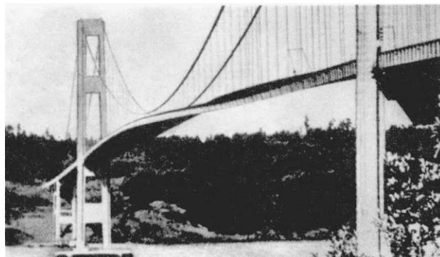
Figure 7: Collapse of Tacoma Bridge
